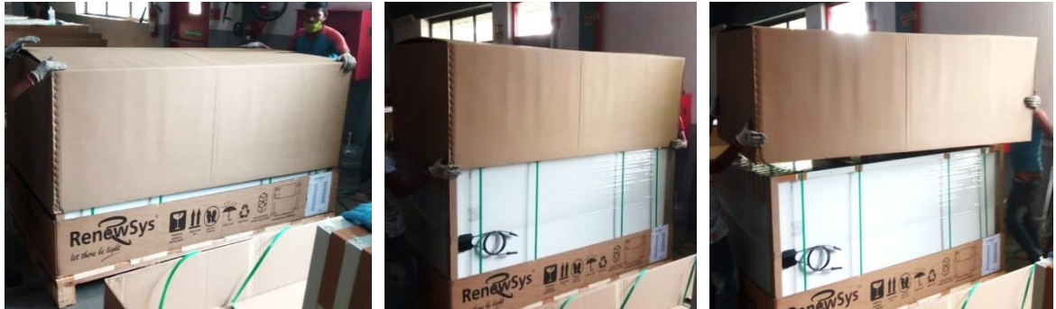
Fig: Opening the lid of Standard Packing box - 2
